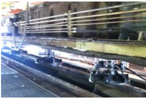
under lowering conveyor
